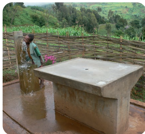
Southern Ethiopia: Clean water well installed by the NGO Inter Aide
