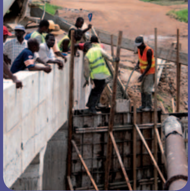
Drain construction © Thomas de Gubernatis
