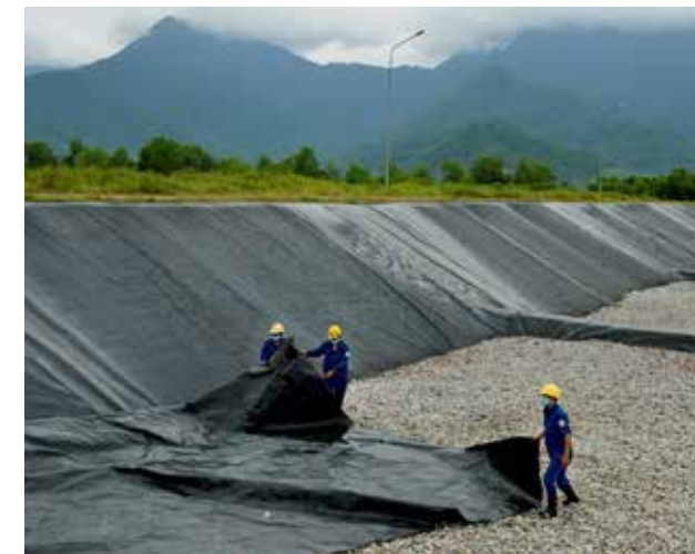
Figure 16: Installation of the waterproof tarpaulin on the new cell at the Lọc Thủy landfill. Lãng Cô, Vietnam.
