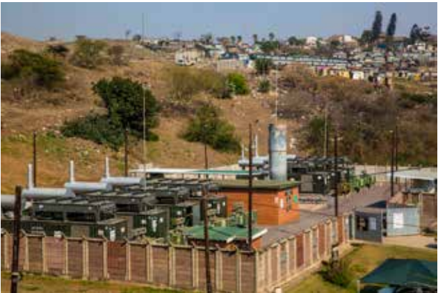
Figure 27: Overview of the eThekweni power plant, which recovers the methane formed by the fermentation of waste and uses it to produce electricity. Durban, South Africa.
