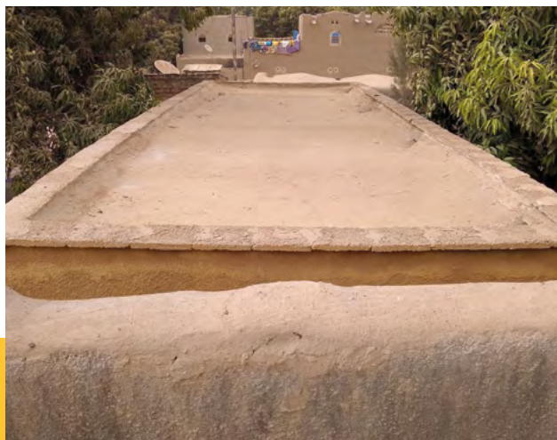
Example of roof terrace.
