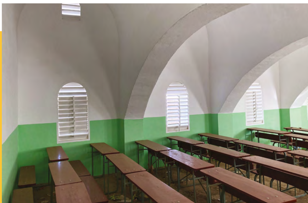
Open space between the vaults thanks to solid concrete block arches for a classroom with a length of 9m50 and a width of 6m50.
