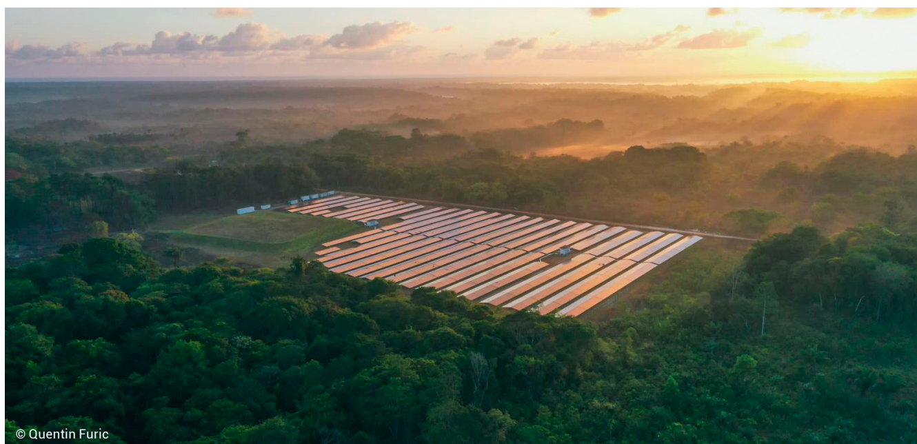
Sinnamary solar power plant, French Guyana
