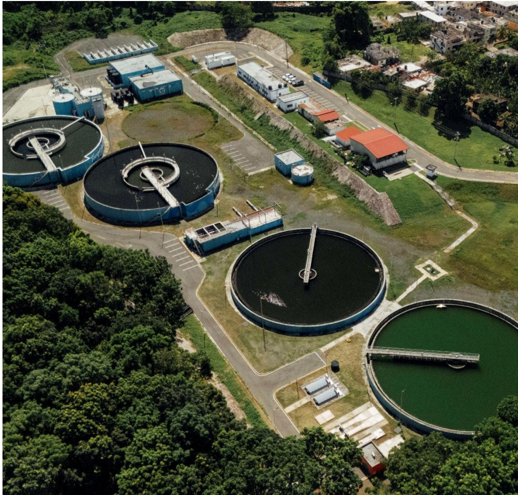
Wastewater treatment plant in Dominican Republic, part of a sanitation and sewerage infrastructure improvement project financed by AFD.
