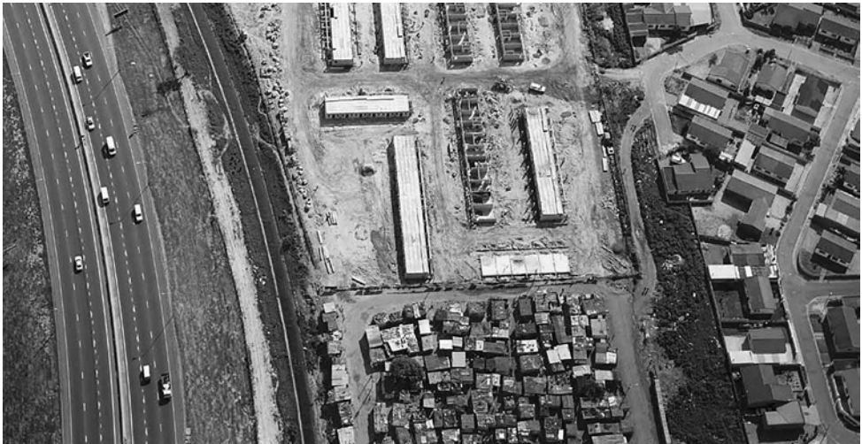
Figure 2: The N2 Gateway project underway in Cape Town, 2005 (photograph by City of Cape Town, with permission)
